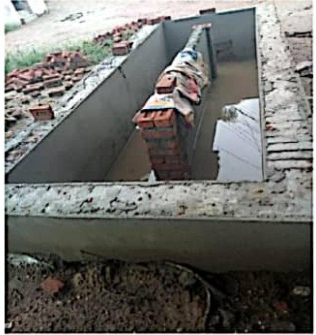
POND 1 AFTER (DESILTING CHAMBER)
